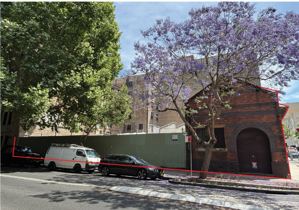
Figure 5. Looking west at the Mountain Street frontage
