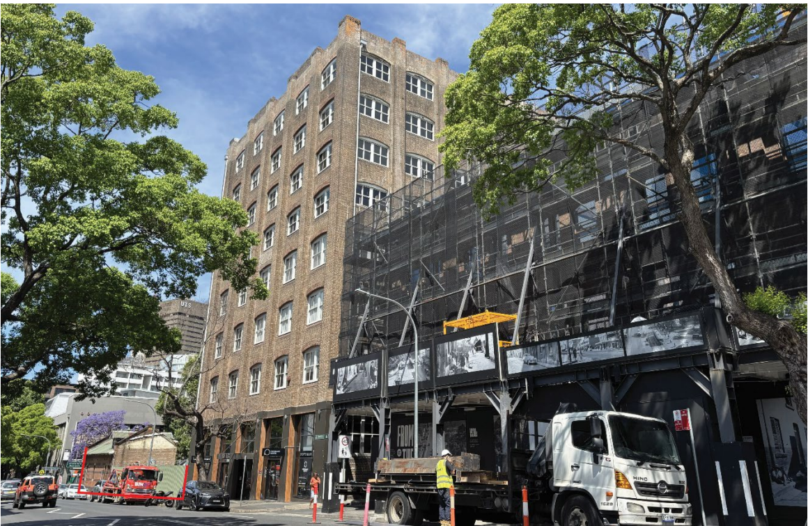
Figure 7. Looking south-east down Smail Street towards the site
