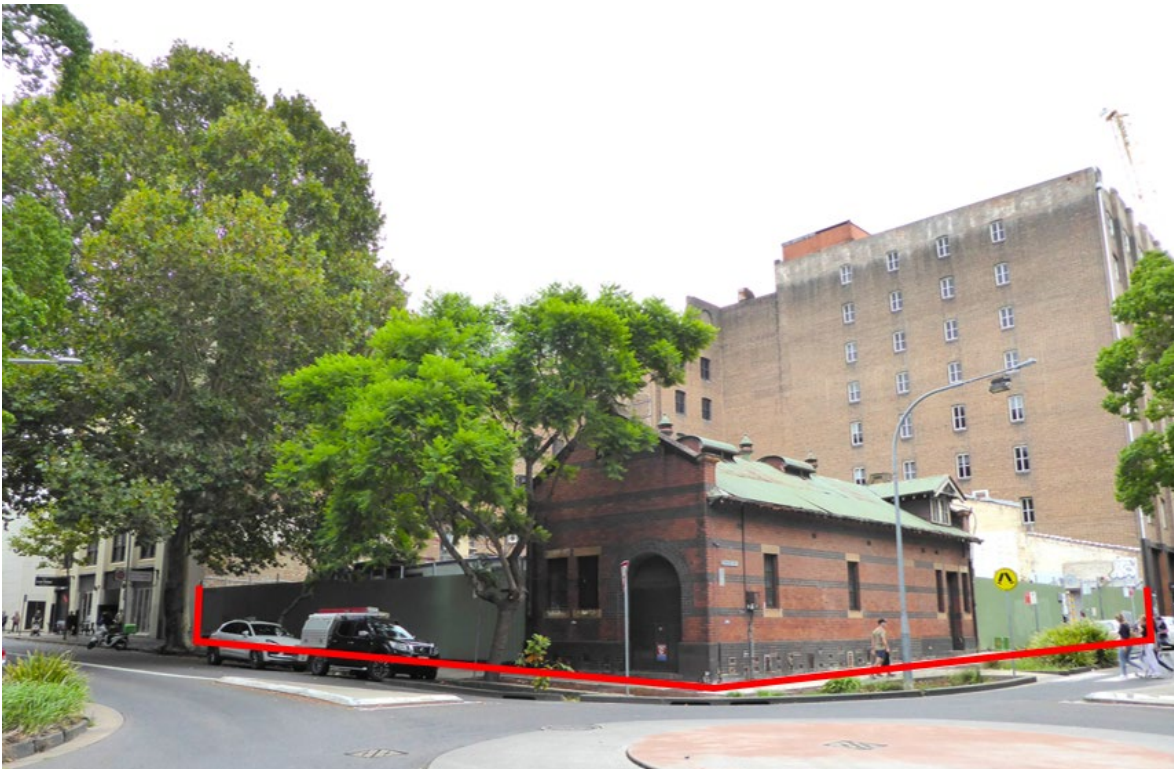
Figure 3. Subject site outlined in red, looking south-west at corner of Mountain and Smail Streets
